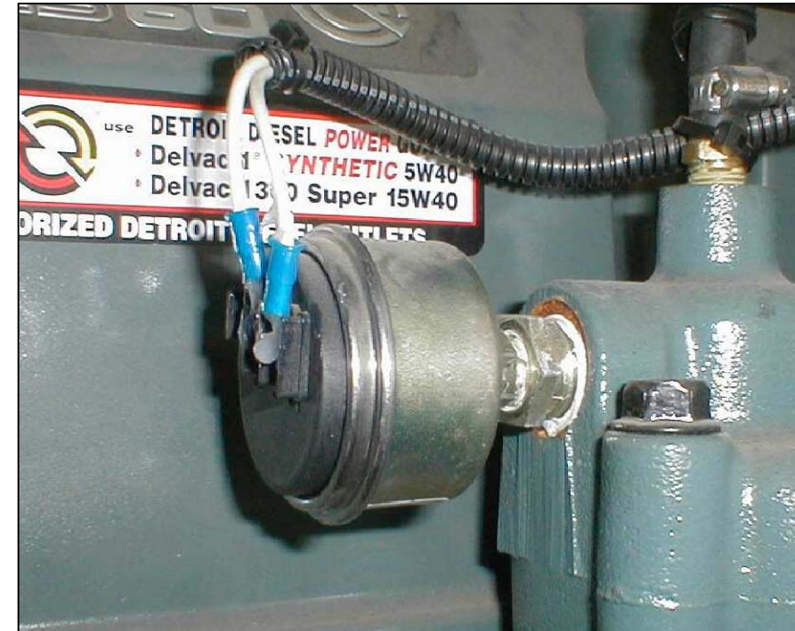
ADDED TEMPERATURE SWITCH
